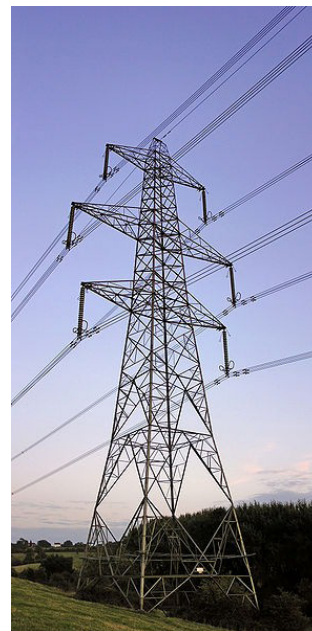
Aluminum cables for electric power transmission
