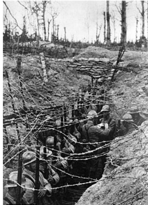
Fig. 1.14 Trenches dug in World War I
