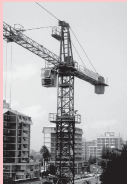
Construction site in Addis Ababa
