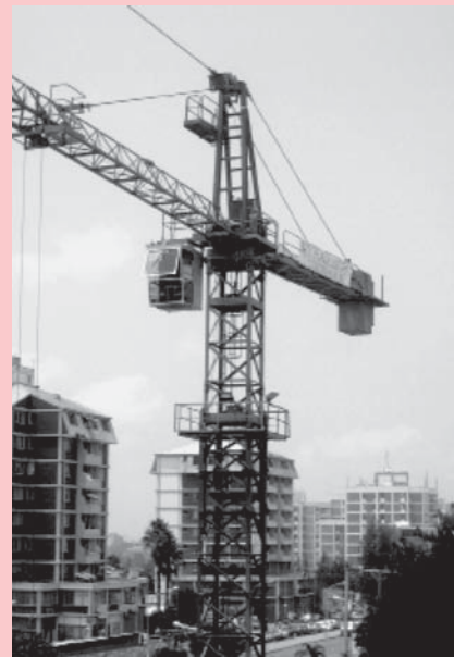
Construction site in Addis Ababa
