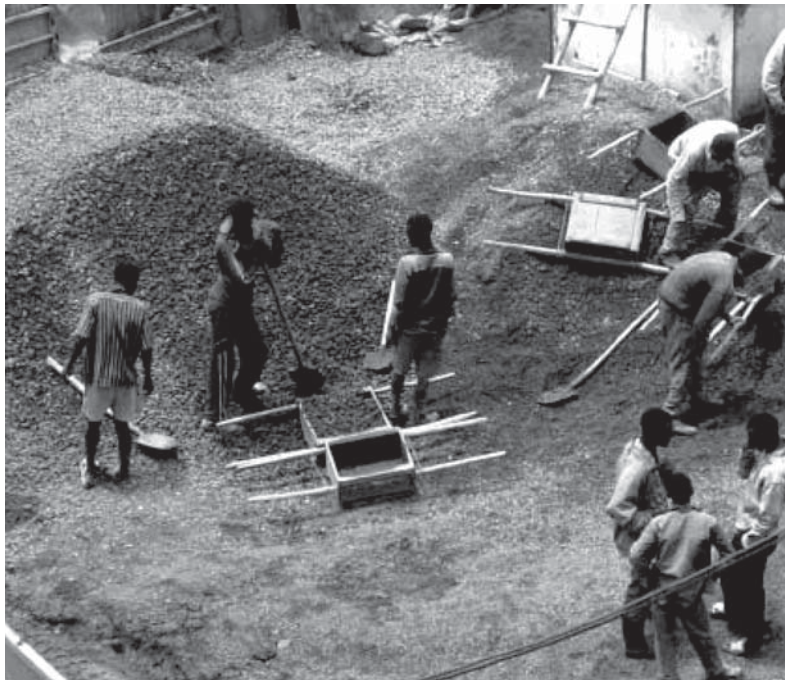
A group of blue collar workers on a building site
