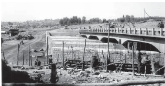
Road built as a result of co-operation with other countries
