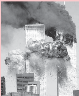
The twin towers in New York destroyed by terrorists in 2001
