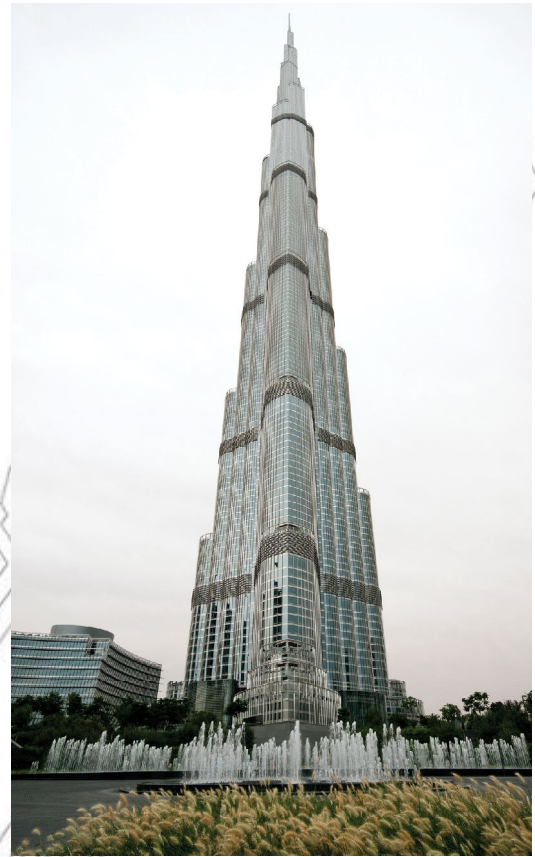
At 828 m in height, Burj Khalifa in Dubai is the tallest building in the world. It has offices, shopping malls, nine hotels, over 30,000 flats and homes, and the world's highest mosque and highest swimming pool.
