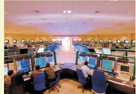
Fig. 1.19: An air traffic control system
