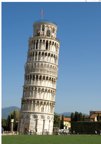
Figure 2.24 The Leaning Tower of Pisa
