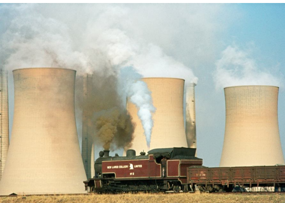
Figure 4.40 An example of a coal-fired power station
