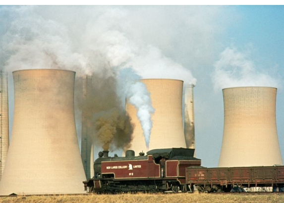
Figure 4.40 An example of a coal-fired power station
