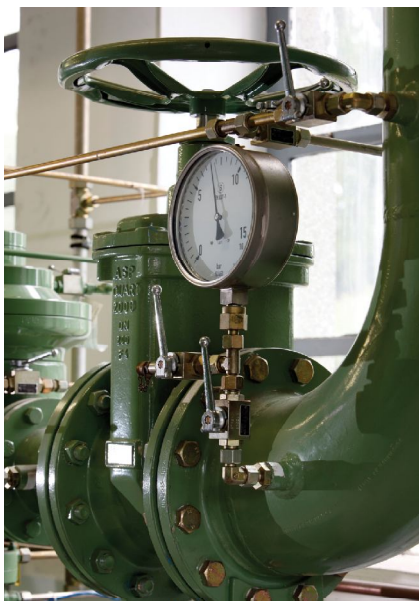
Figure 6.42 A manometer being used
