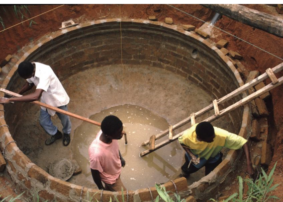
Figure 1.12 Biogas generators like this have made an enormous difference to many families by producing cheap and readily available fuel.
