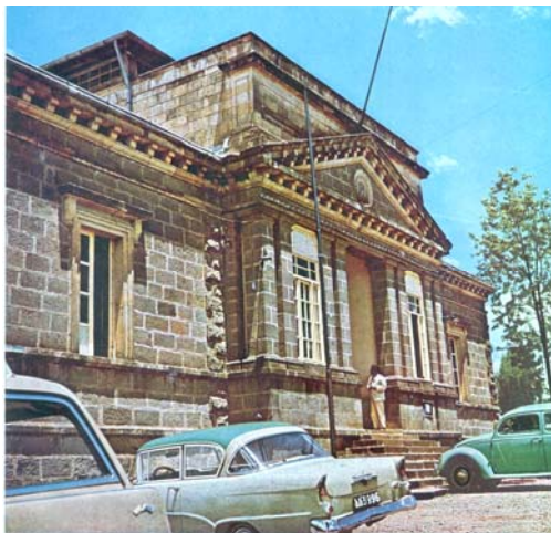
Figure 3.9 Bank of Abyssinia
